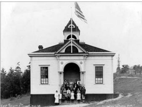
East Seattle School District School ("the little white schoolhouse"), Mercer Island, 1909
