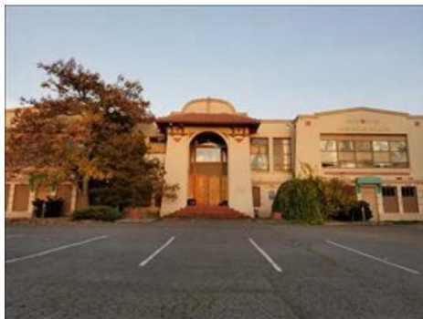
East Seattle School north elevation, Mercer Island, 2018
