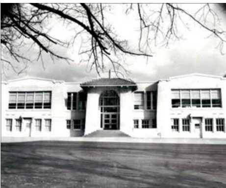
West face, main entrance, East Seattle School, Mercer Island, n.d.
