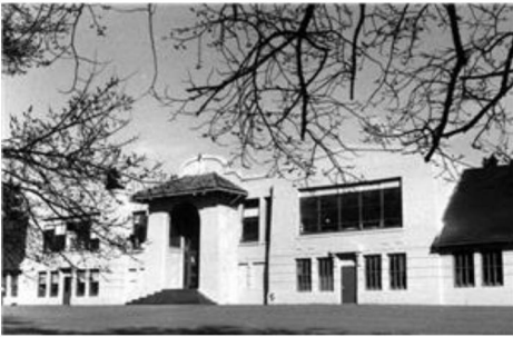
East Seattle School, west side, Mercer Island, n.d.
